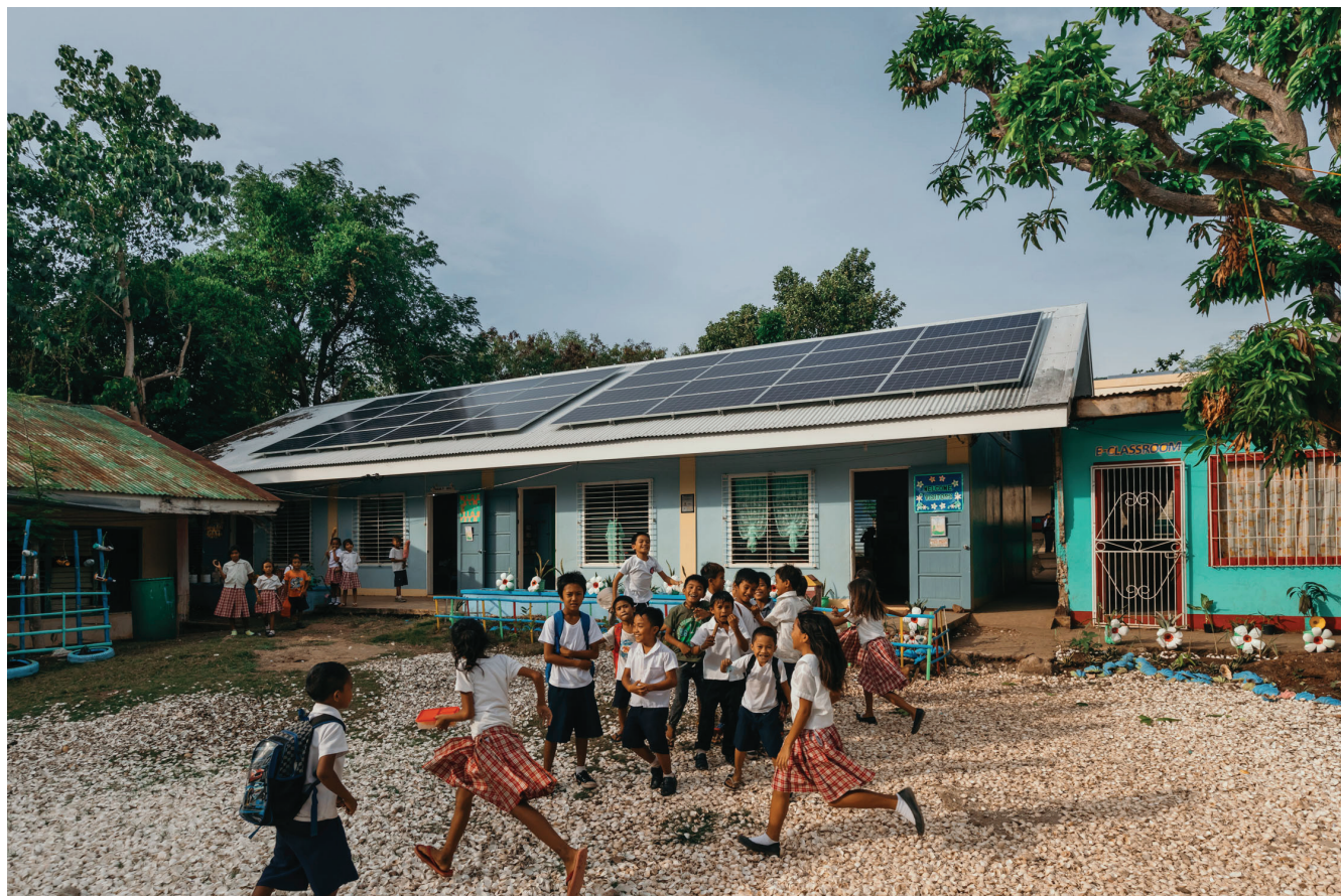
Pilot project for solar electrification of schools - Hilotongan Integrated School in the municipality of Bantayan
